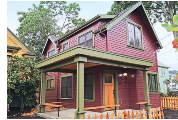
▶ An ATTACHED ADU connects to an existing house, typically through the construction of an addition along the home’s side or rear. Such units can have a separate or shared entrance.
